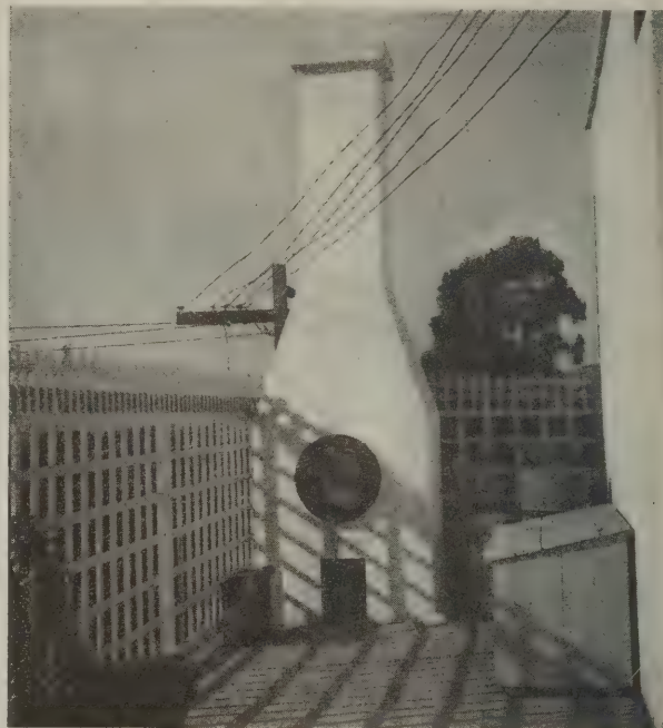
INCINERATOR AT REAR OF COURT. A NEW AND IMPORTANT FEATURE.
